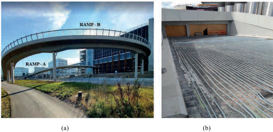
Fig. 3. a) Ramp A and ramp B with HRS in Ingolstadt and b) laying pattern of heating pipes during installation.
