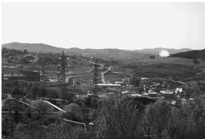
Fig. 4. Dry-steam plant, installations and transmission lines at Larderello (Italy) with a total exploited area of around 250 \text{km}^2 .
