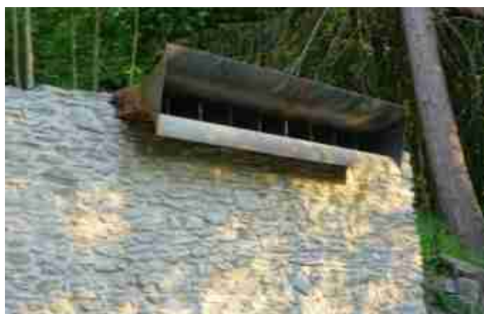
Fig. An object with a "mouth-like" steel structure was installed to prevent predators from catching bats in the FFH site (Flora-Fauna Habitat) at Büchenberg (Saxony-Anhalt, Germany).
